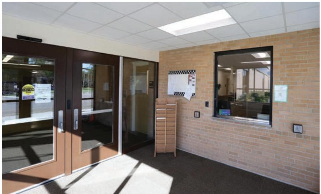
*Limiting access is one element of safe school planning. Increasingly, schools are adding a layer of security for office staff by incorporating a transaction window, sometimes with bullet-resistant glazing.*
